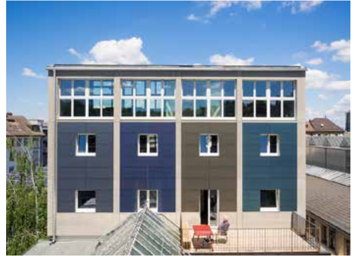
Kohlesilo CH-Basel, Solvatec AG
