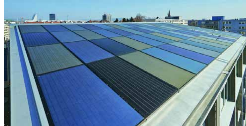
Kohlesilo CH-Basel, Solvatec AG
